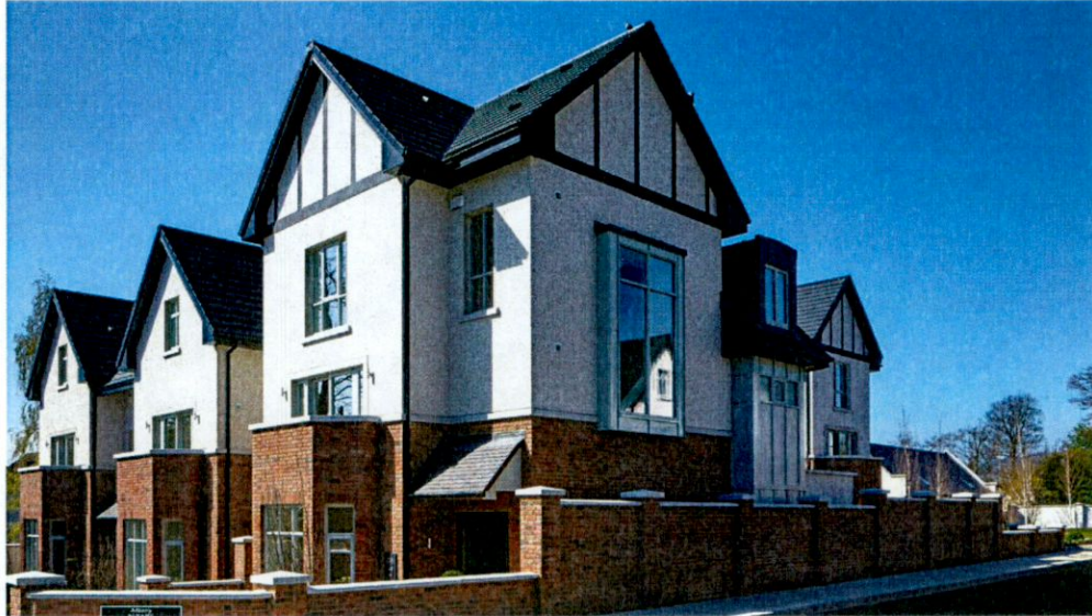
Figure – 3 storey Houses - Source – Google Images
