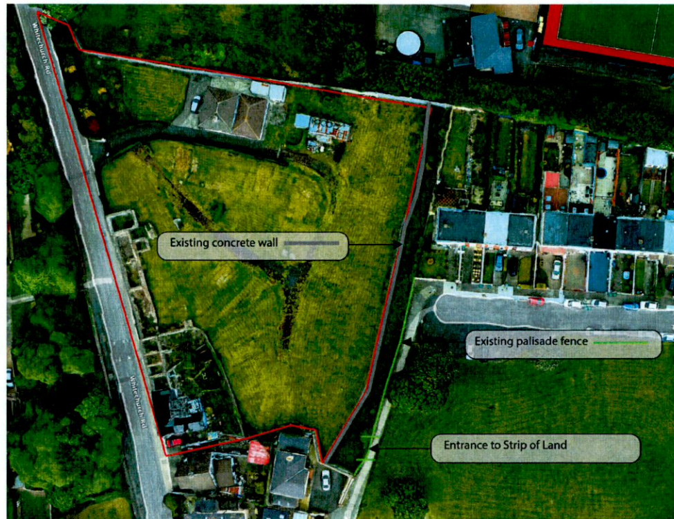
Figure 12 - Location of existin concrete wall and paliside fence prepared by Brock McClure
