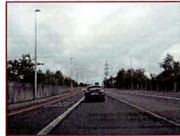
FIGURE 2-2: R136 TRAVELLING SOUTHBOUND
