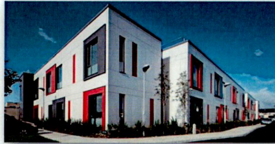
Figure 4.3 – Ennis Hospital – Cladding Panel system
