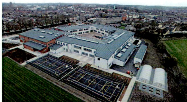
Figure 4.2 – Aerial view of a new school complex
