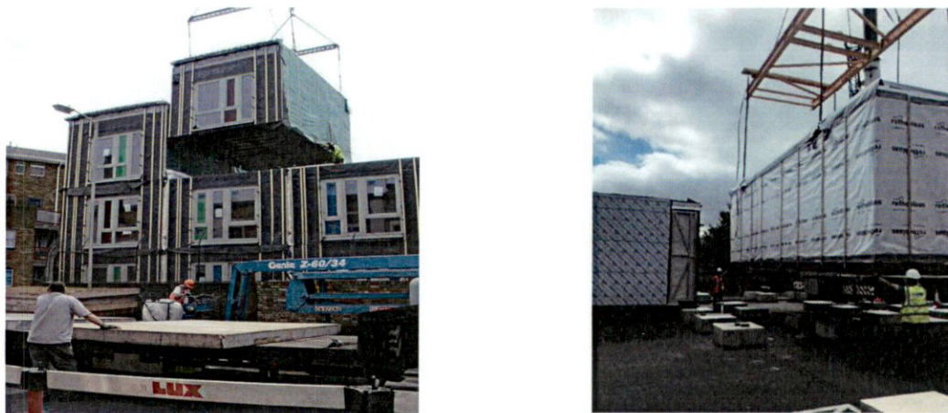
Figure 3.4 – Modules delivered to site
