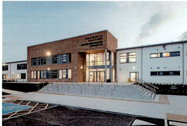
Figure 4.1 – New School Building – Carrigaline, Co. Cork
