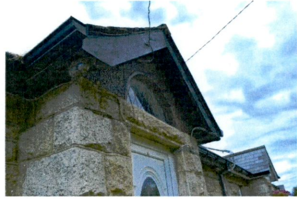
-Rear Elevation, No.626 Whitechurch Road
