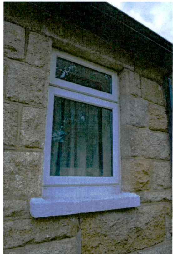
-Example of UPVC window to be replaced
