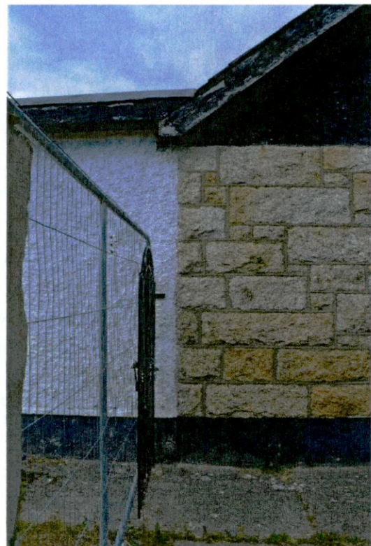
-Junction of existing cottage and existing rear extension
