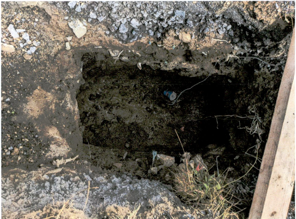
#06 – Day after 3 rd fill, 30 th July 2022.
