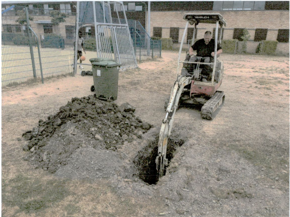
#01 – Trial pit excavation for percolation test – 27 th July 2022.
