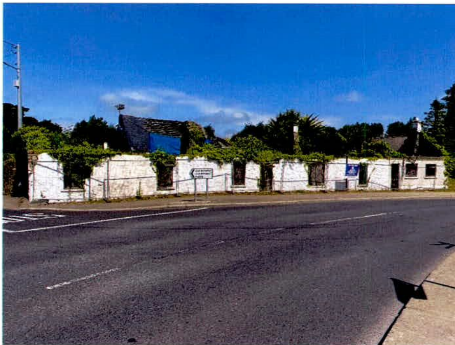
Plate 2. View of NIAH 11212011 looking north.
