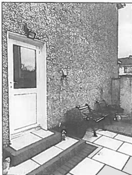
Fig. 2 - Existing Access Door to Garden on West Elevation
