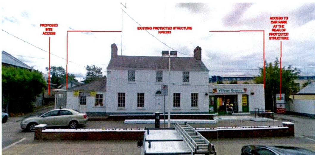
Existing Protected Structure, proposed site access and access to car park at the rear.
