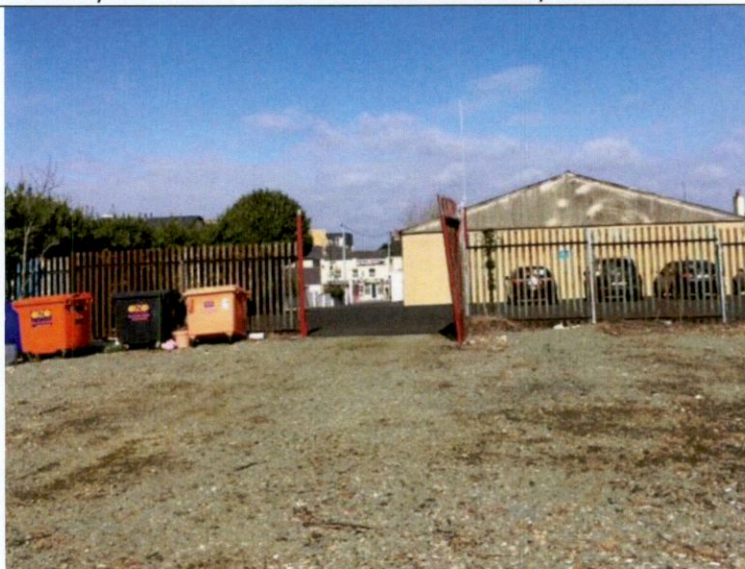
2. View of commercial unit from rear, and dividing fence and gate.
