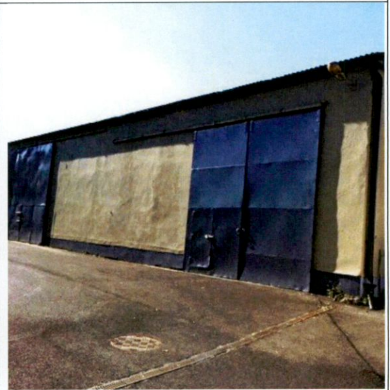
3. Side wall of commercial unit. To be removed.
