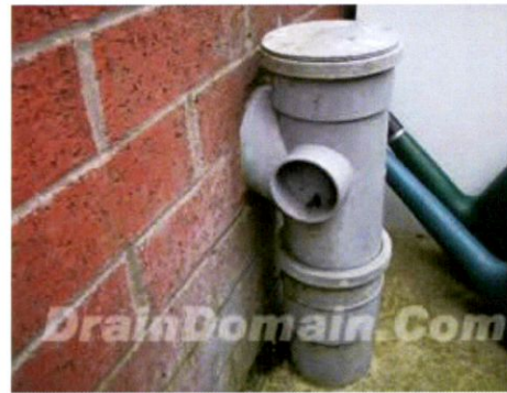
Pipesnug Seal (or similar) - External Wall Penetration
