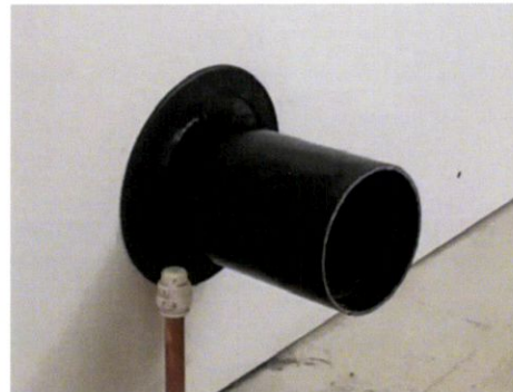
Example Pipe Protection (1)
