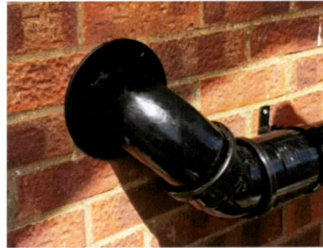
Pipesnug Seal (or similar) - Internal Wall Penetration
