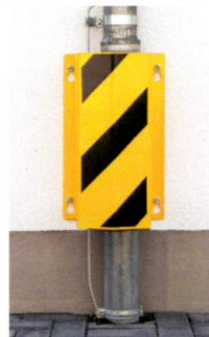
Example Pipe Protection (2)
