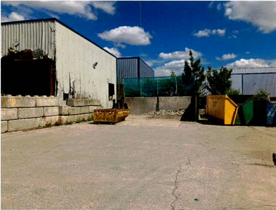
Figure 10.17: Rear of existing buildings (view from yard area facing east)
