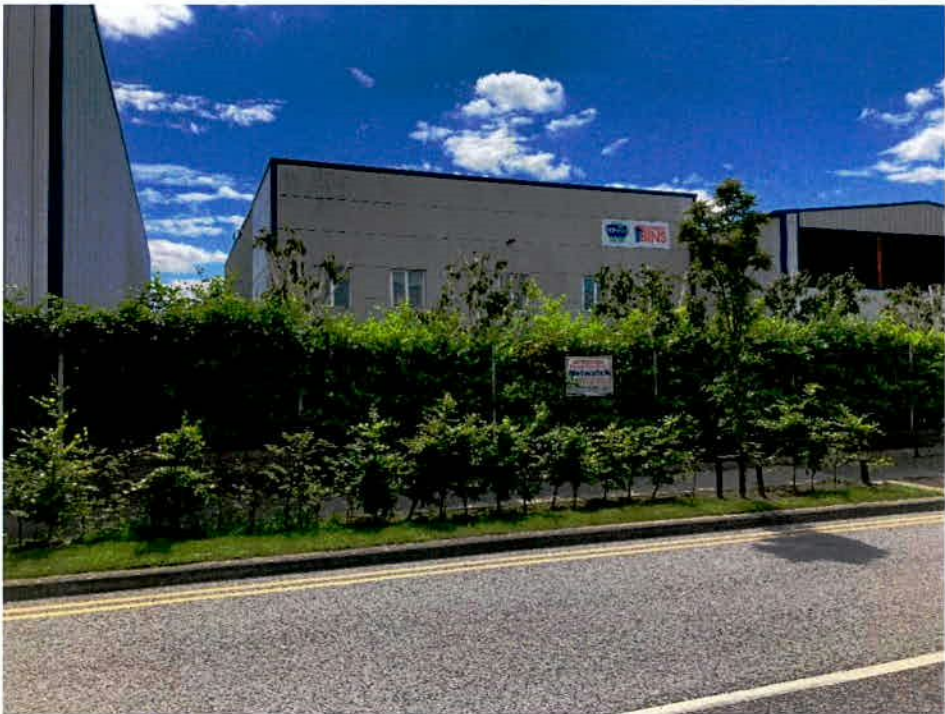
Figure 10.15: Existing buildings (view from Grants Crescent facing south)
