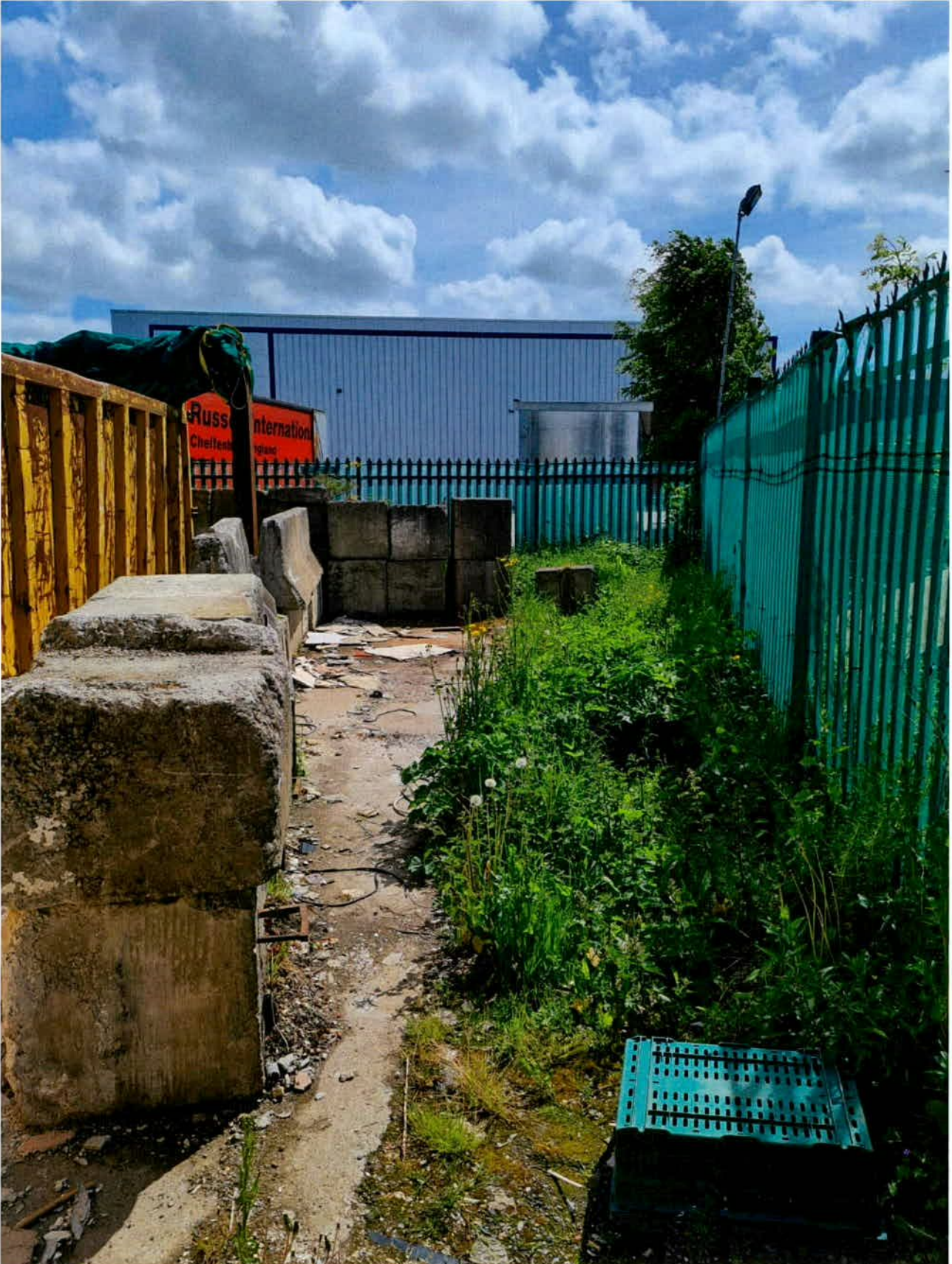
Plate 6: Section of recolonised bare ground habitat at southern end of the site (view facing east)
