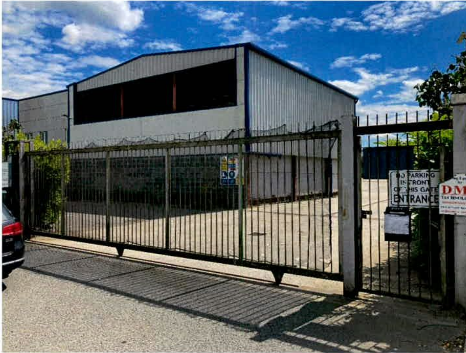
Figure 10.13: Existing buildings (view from site entrance facing southeast)
