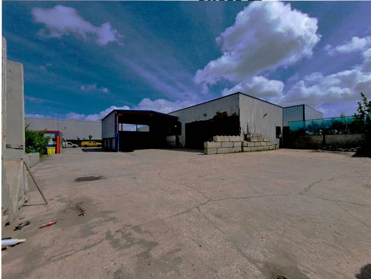
Plate 4: Concrete yard behind existing buildings (view facing north)
