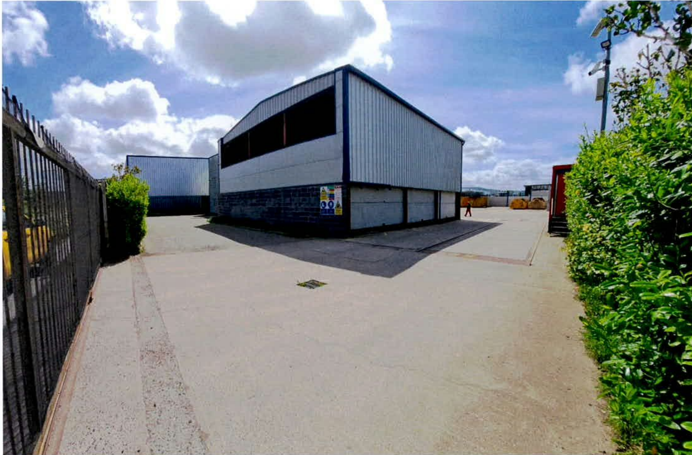
Plate 1: Site from the access gate
