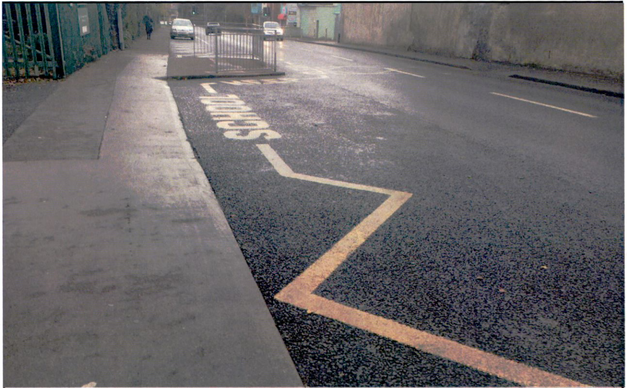
Photograph 3 – Existing road markings at the school access
