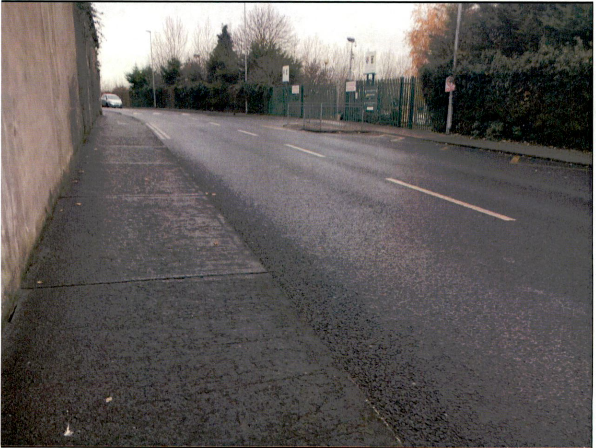
Photograph 5 – Existing gated school access
