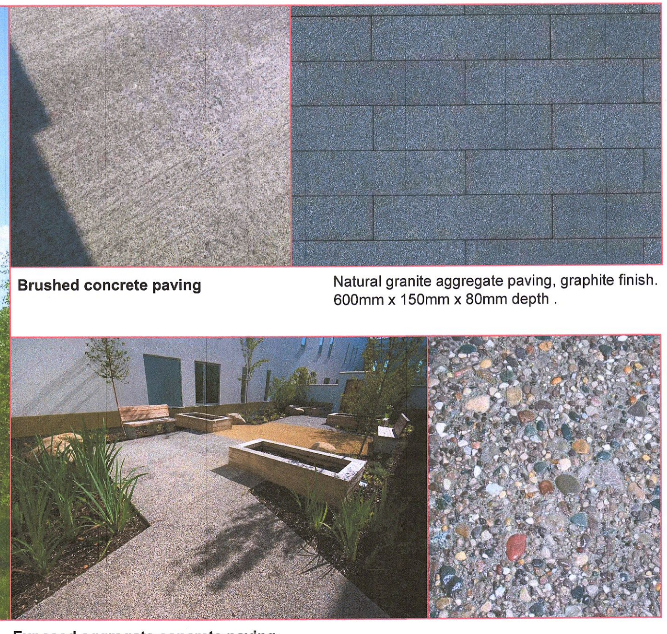
Brushed concrete paving Natural granite aggregate paving, graphite finish. 600mm x 150mm x 80mm depth. Exposed aggregate concrete paving
