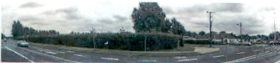
Fig 3 – View of pedestrian route at Northern boundary along New Nangor Road
