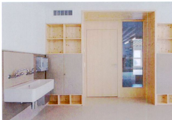
▲ Plywood Wall Cladding
