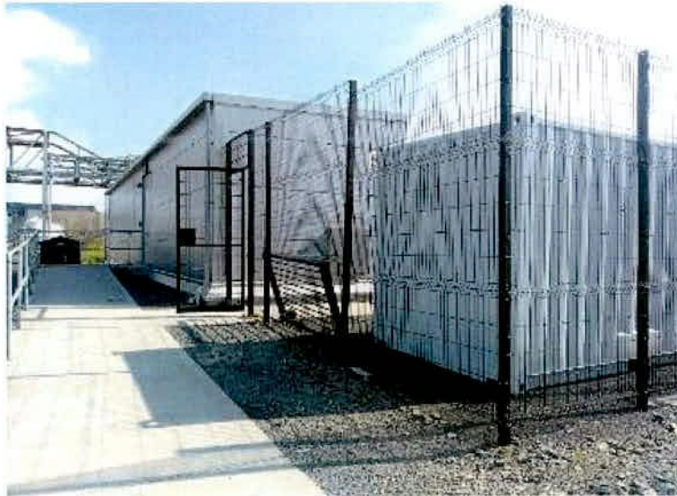
Existing Paladin weldmesh black fencing on site - Proposed fencing to match
