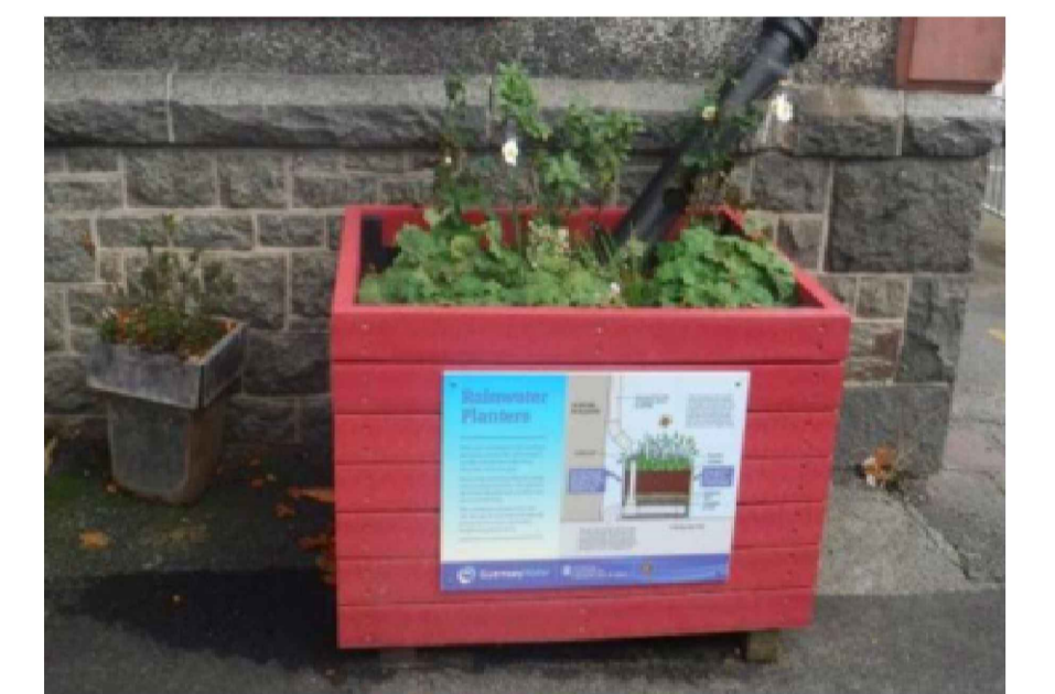
IMAGE EXAMPLE OF RAIN GARDEN PLANTER BOX DETAIL (FROM SOUTH DUBLIN COUNTY COUNCIL PUBLICATION, A HOUSEHOLDERS GUIDE TO SuDS)
