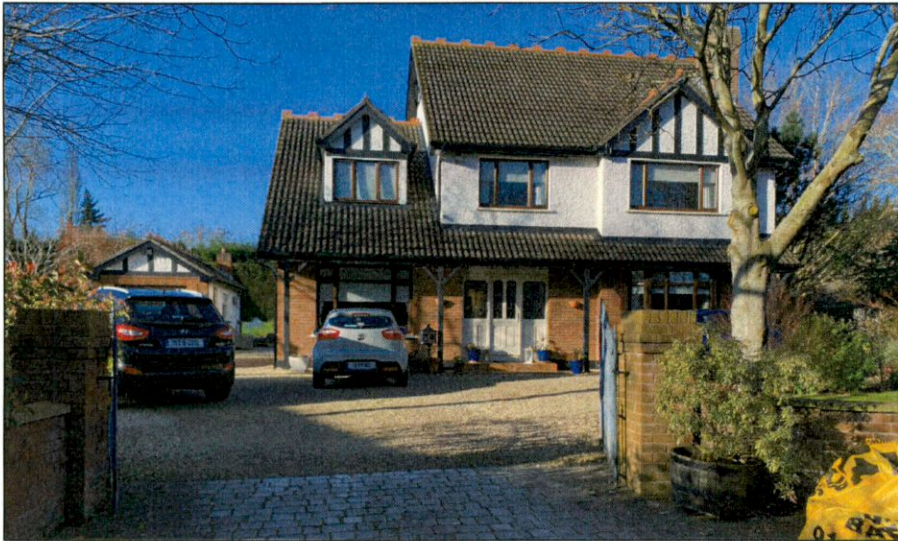
Front elevation and garage to be demolished of The Muddies from private laneway
