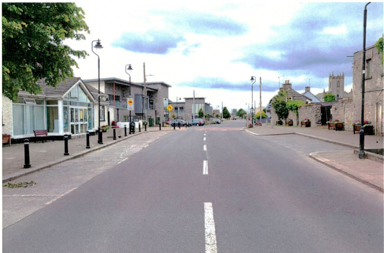
Figure 3.4: Forward visibility of eastbound vehicle on approach to development access (source: SRC, June 2022)
