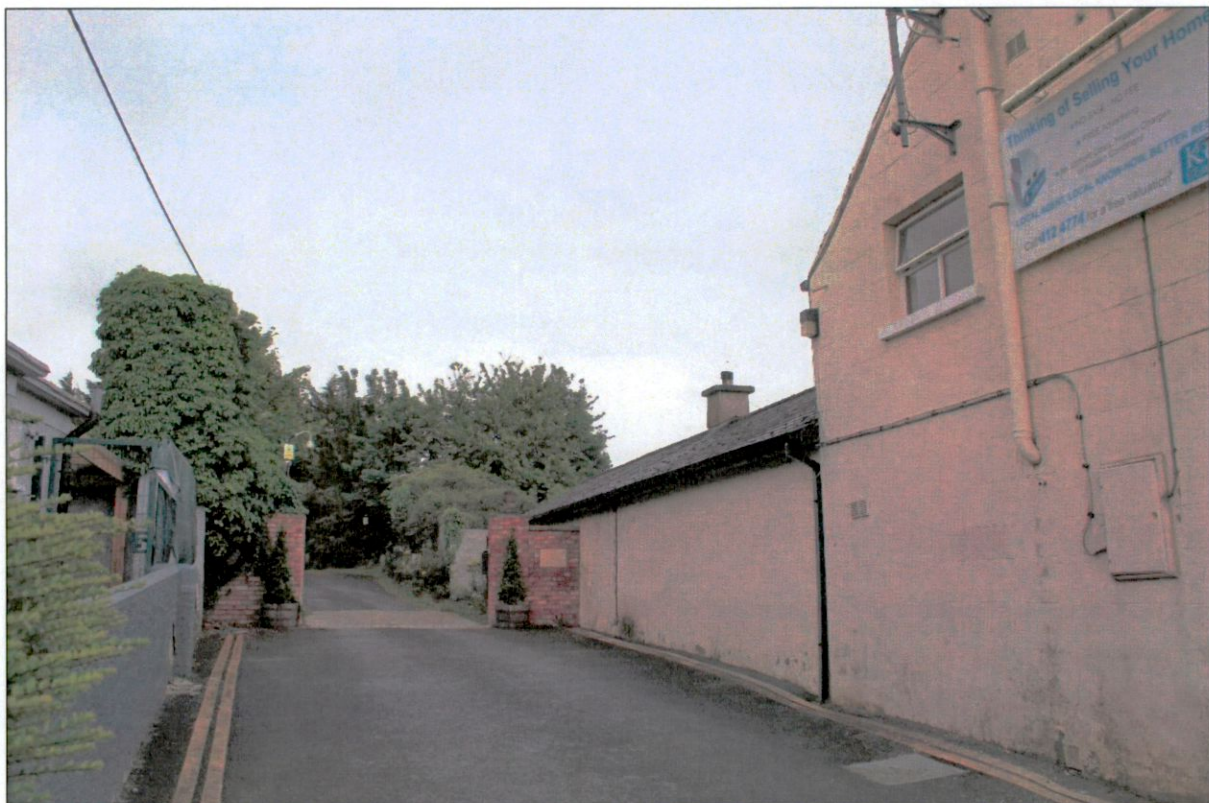
Plate 14: Entirely modern east boundary treatments to north end of site behind Kelly Estates building (east gable of which to right side of photograph). No changes to any existing fabric here as part of present proposals.
