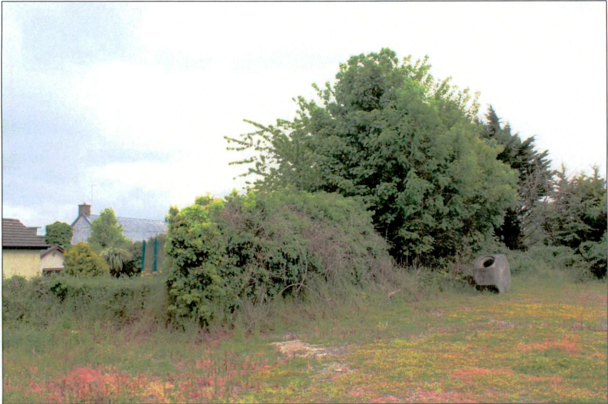
Plate 13: Heavily overgrown boundary wall to rear (south) of garden behind modern L-shaped dwelling which may be remnant of historic brick boundary wall depicted on 25" OS map here. Wall here proposed to be demolished.
