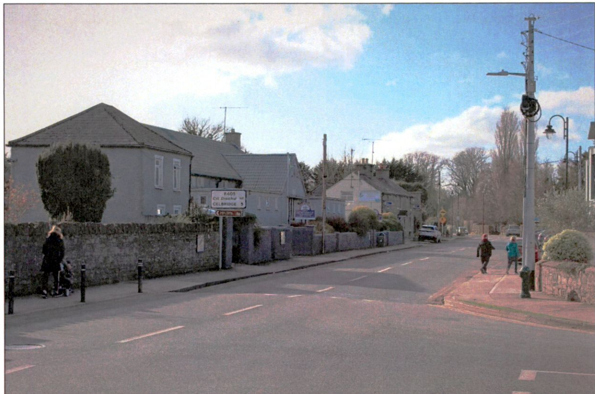
Plate 22: View west along R405 (Kelly Estates building right of centre of photograph) illustrating essentially historic character of streetscape here with strong masonry edge and variety of traditional building forms to south side of street.
