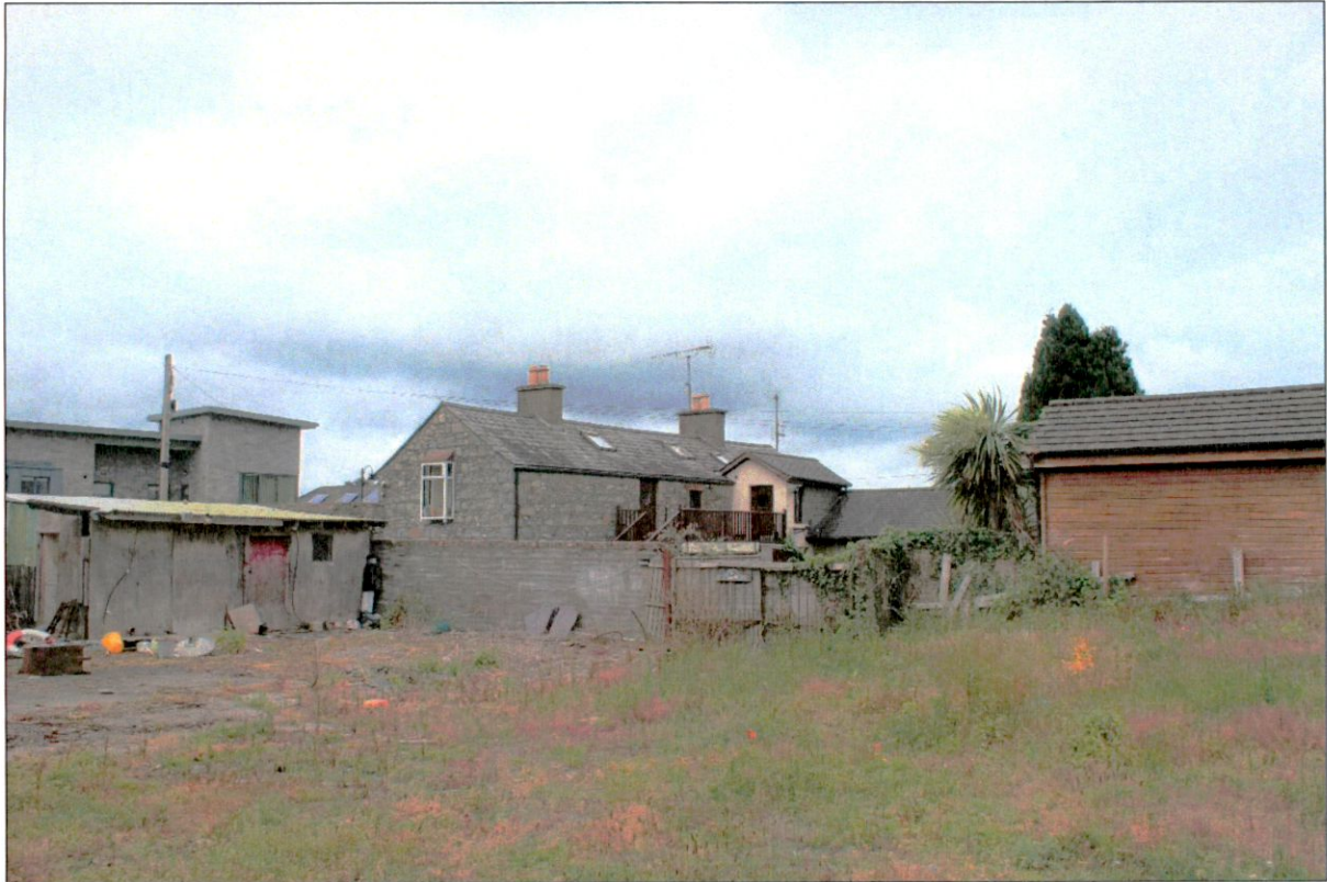
Plate 9: Site interior looking north-east towards Kelly Estates building to be retained.
