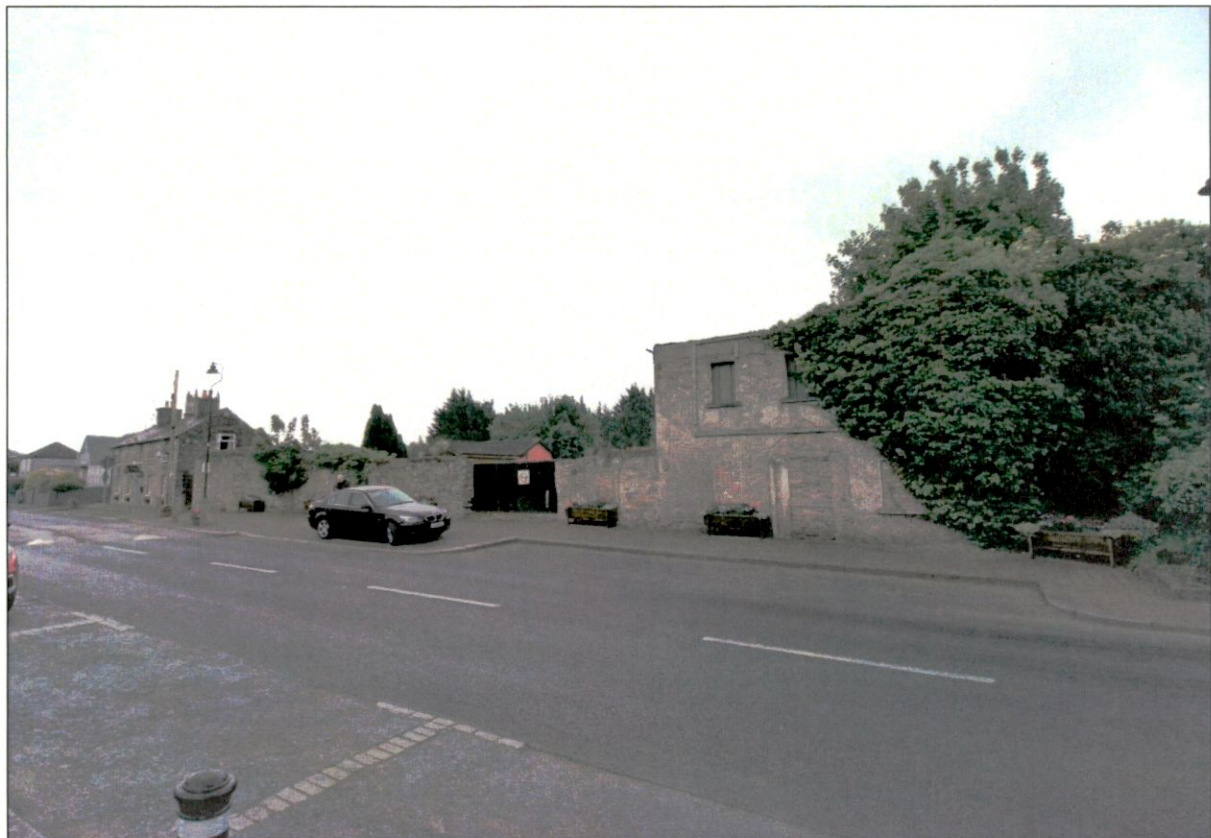
Figure 2: View of site exterior from Main Street looking towards south-east.
