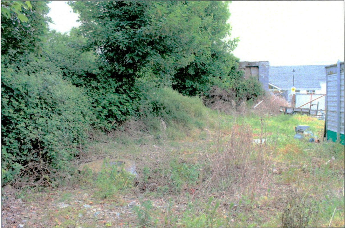
Plate 17: View to north along northern end of western boundary with manhole over confluence of culverted streams flowing from south and east before heading north along western boundary of site.
