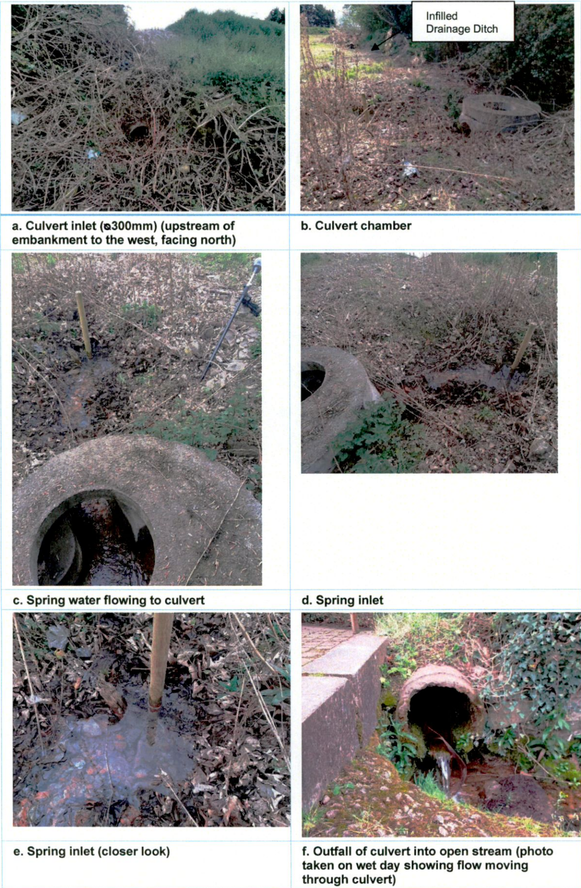
Figure 2-4: Drain features
