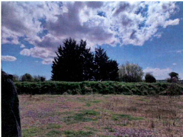
Figure 2-2: Existing earthen embankment (Site looking towards the south)
