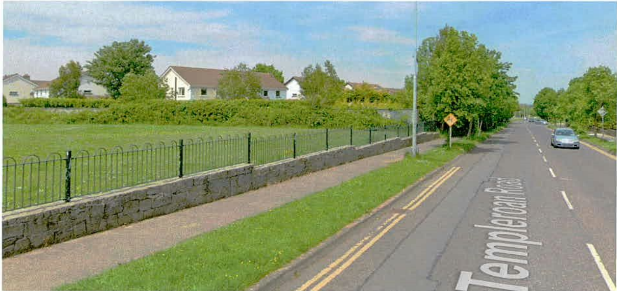
VIEW OF THE SOUTHERN BOUNDARY SHOWING NO 48 WITH BUSHES ALONG THE BOUNDARY TO PROVIDE GARDEN LEVEL PRIVACY AND SECURITY. FIRST FLOOR WINDOWS IN SOUTH AND EAST WILL OVERLOOK THE PUBLIC OPEN SPACE.
