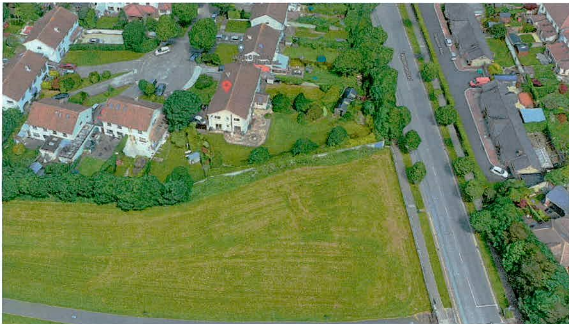
Aerial View of No 48 (Red dot) with No 47 to left (west) and single storey dwellings on Templeroan Road to right (East)
