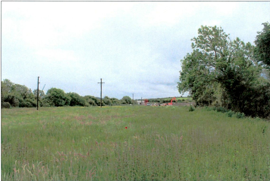
Plate 3: View to south-southeast, showing the southern portion of the proposed development site, which comprises fairly level, dry grassland between two long-established hedgerow boundaries to east (left) and west (right)
