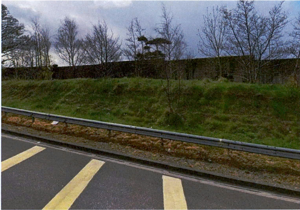
Figure 5: Image From Street level on the M50 N4 Slip Road
