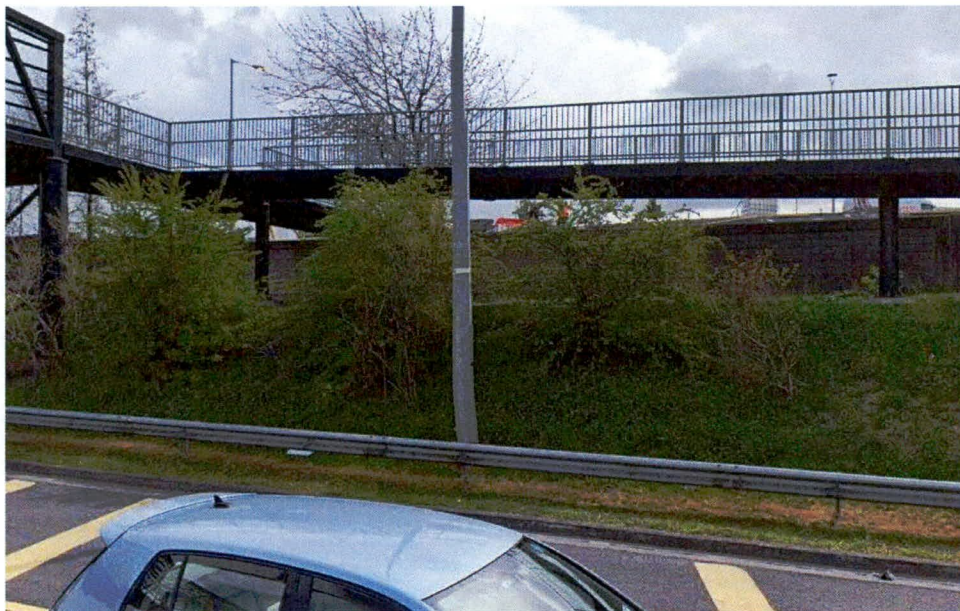
Figure 6: Image From Street Level on the N4
