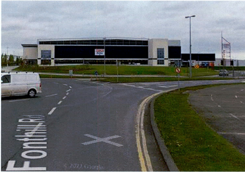
Figure 7: Image From Street Level to the South of the Installation
