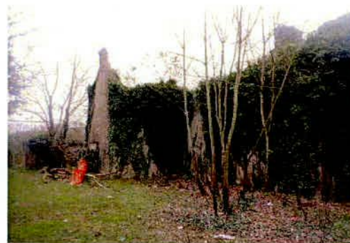
Plate 10 View of rear (west) elevation to Cappagh House, facing southeast
