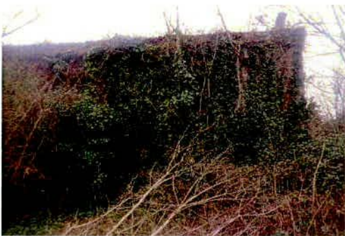
Plate 9 View of front (east) elevation to Cappagh House, facing west
