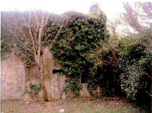
Plate 11 Side (north) elevation of rear block, facing south
