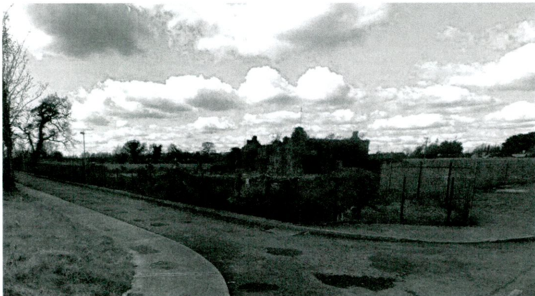
Figure 4 : Ruin of Cappagh House.
