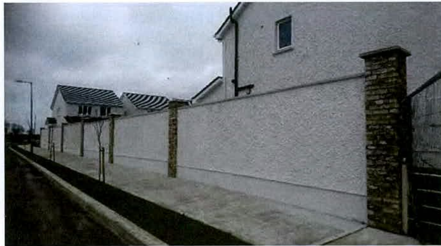
Dash & Brick Pier
