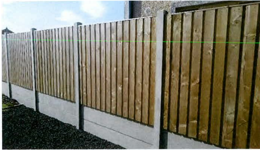
Concrete Post & Wooden Panel Fence
