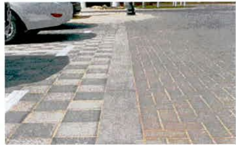
Flush Slipform Concrete Kerb
