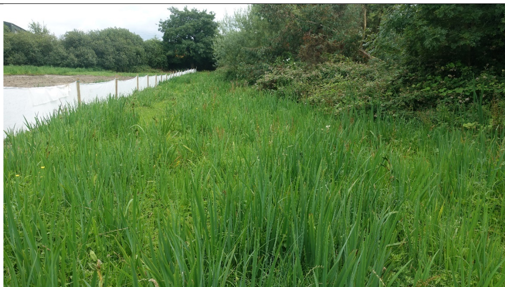
Silt fence from the river showing correct set backs.
