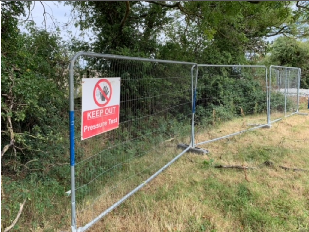
Site fencing and No Entry signage Site side
