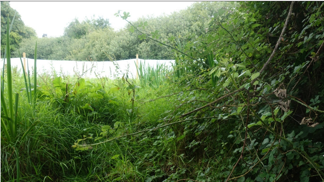
Silt fencing viewed from river
