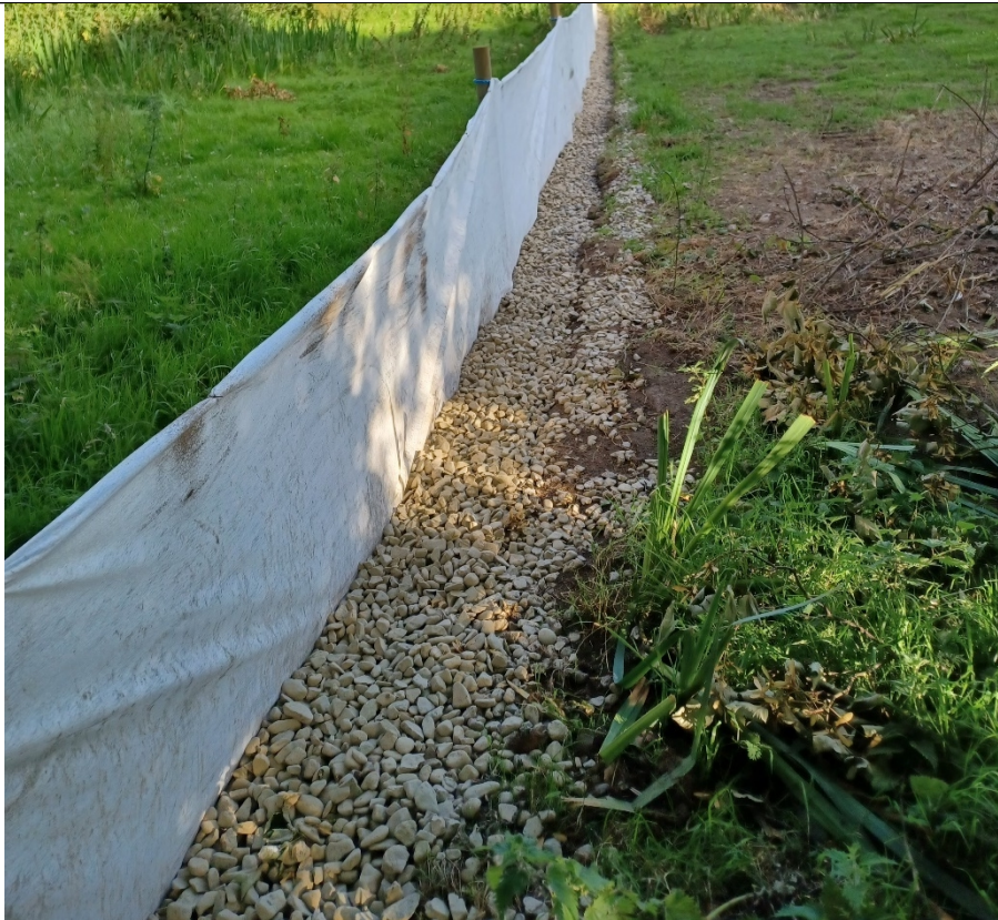
Silt fencing installation
