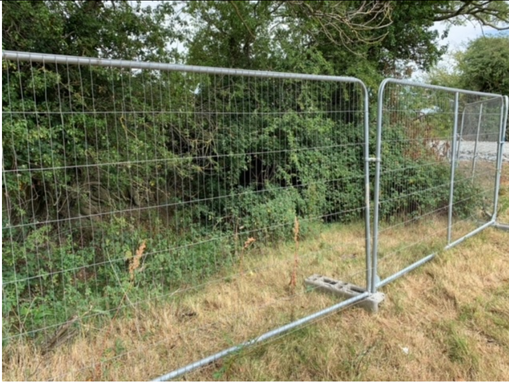
Tree protection fencing at site entrance (site side)
