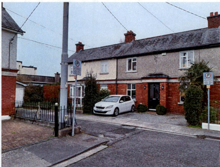
Image 05 – View of vehicular entrances to neighbouring properties
