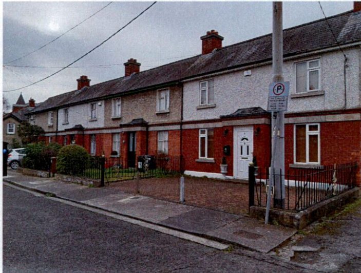
Image 04 – View of vehicular entrances to neighbouring properties
