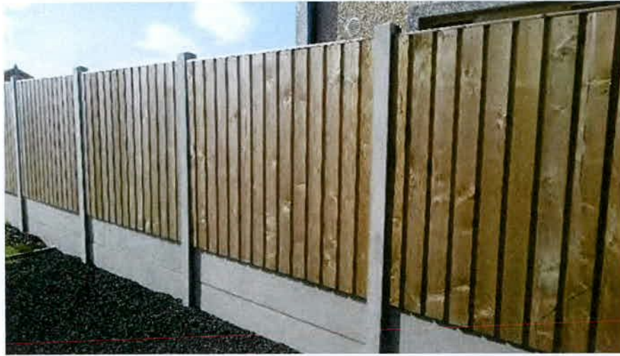
Concrete Post & Wooden Panel Fence
