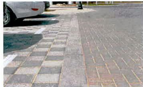
Flush Slipform Concrete Kerb
