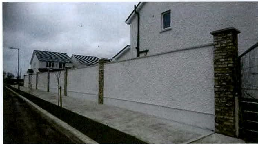
Dash & Brick Pier
