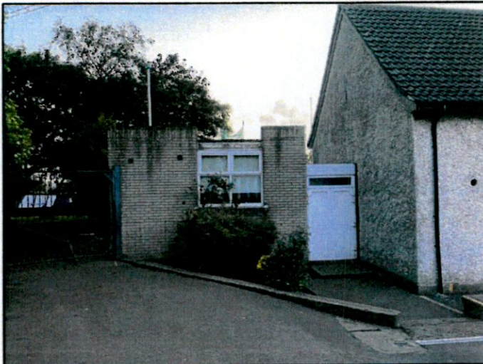
Plate 2 Building to be demolished and location of proposed extension
