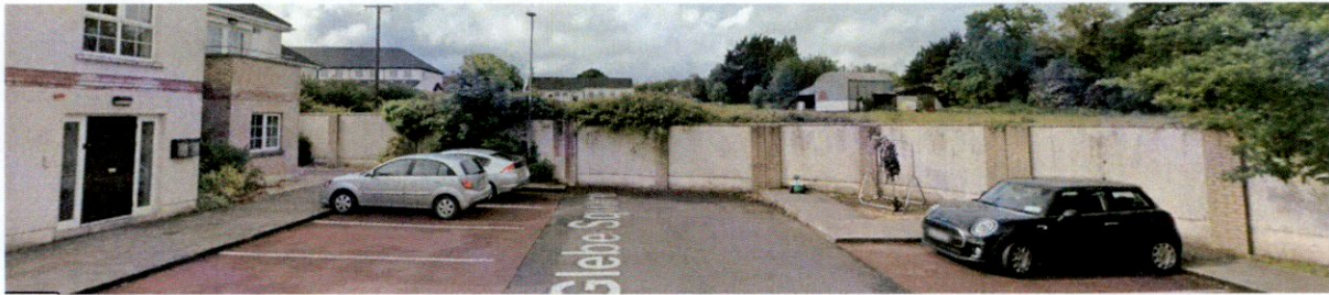
Boundary Wall at end of Road 4 Glebe Square.
