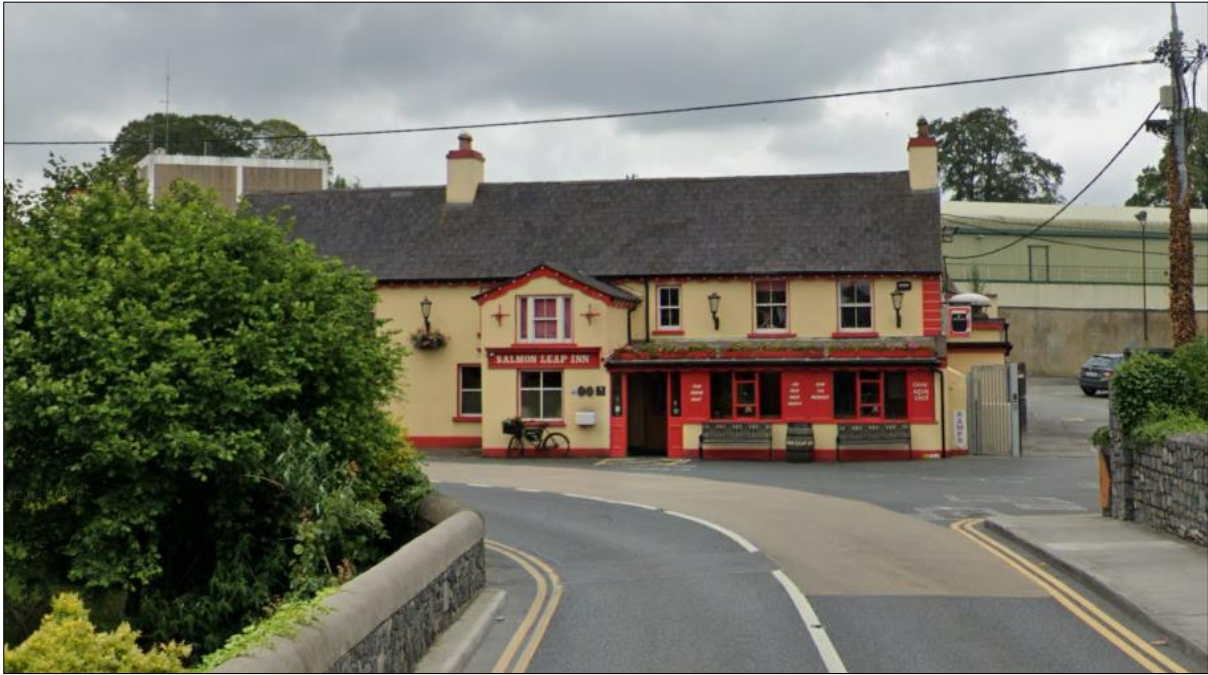
Plate 5: Salmon Leap Public Inn (RPS: 009) with existing WTP infrastructure visible to rear.
