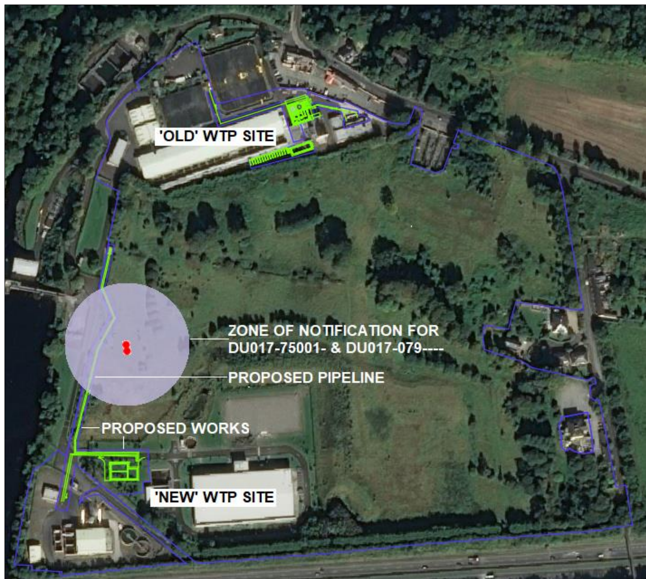
Figure 2: Aerial overview of the existing Leixlip WTP sites with proposed developments and relevant archaeological area indicated (Source: Bing Maps)
