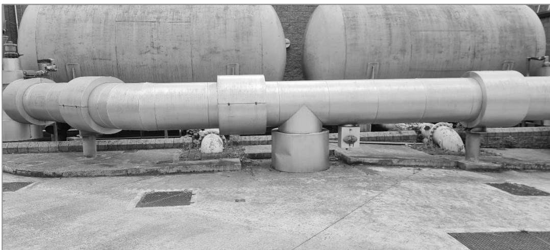
Existing Site Pipe work
