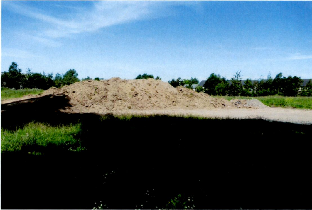
FIGURE 8. SPOIL AND BARE GROUND ED2 ON SITE, WITH AMENITY GRASSLAND GA2 PRESENT WITHIN THE FOREGROUND – PHOTO TAKEN 20 TH JUNE 2022
