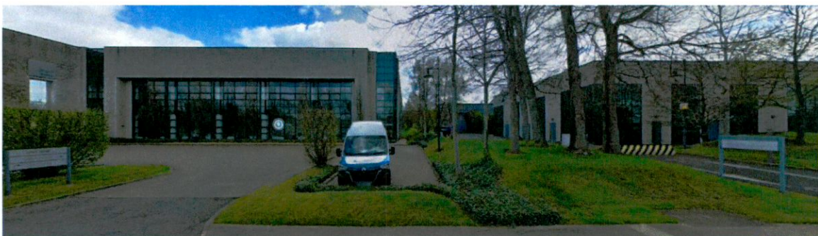
Existing facilities to the east side of the the subject site.
