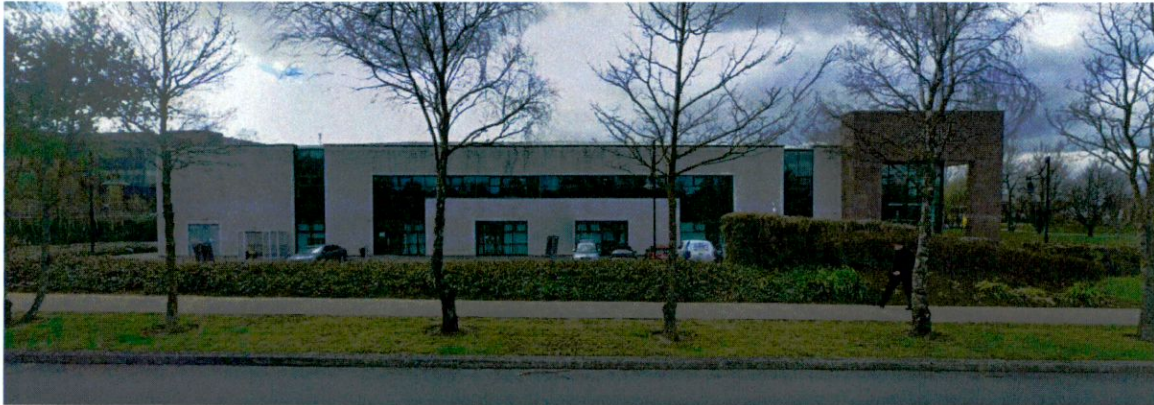
Existing Electronic Facility directly to south of subject site.
