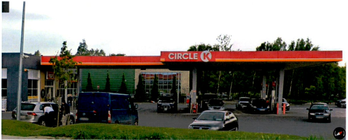
Figure 5: Existing service station fuel forecourt and amenity building
