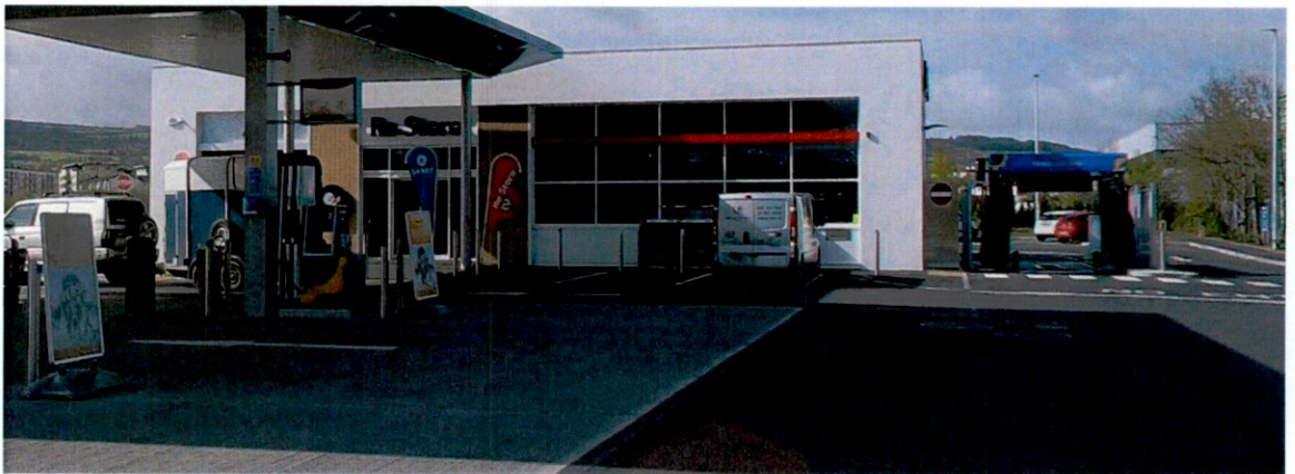
Figure 6: Existing service station amenity building
