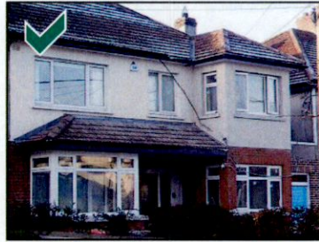
A well designed front and side extension that reflects the character and design details of the original house.
