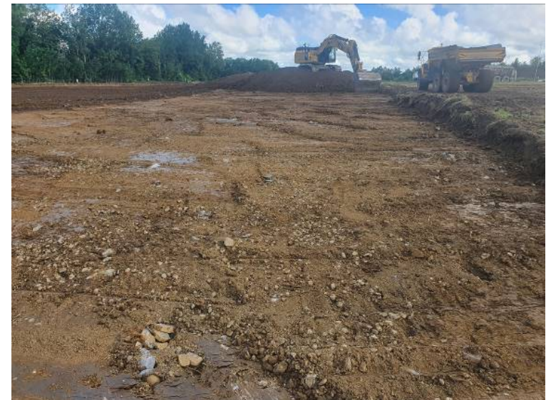
Plate 8 Topsoil stripping, facing north.
