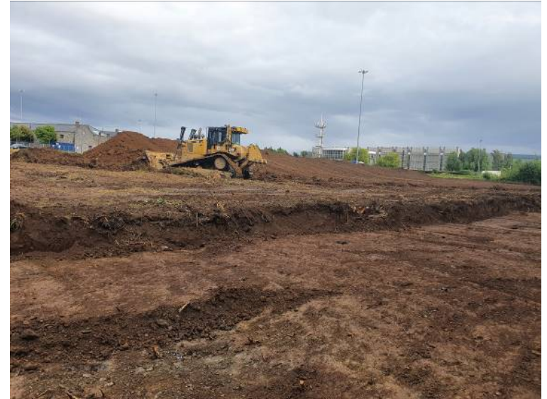
Plate 6 Topsoil stripping, facing southeast
