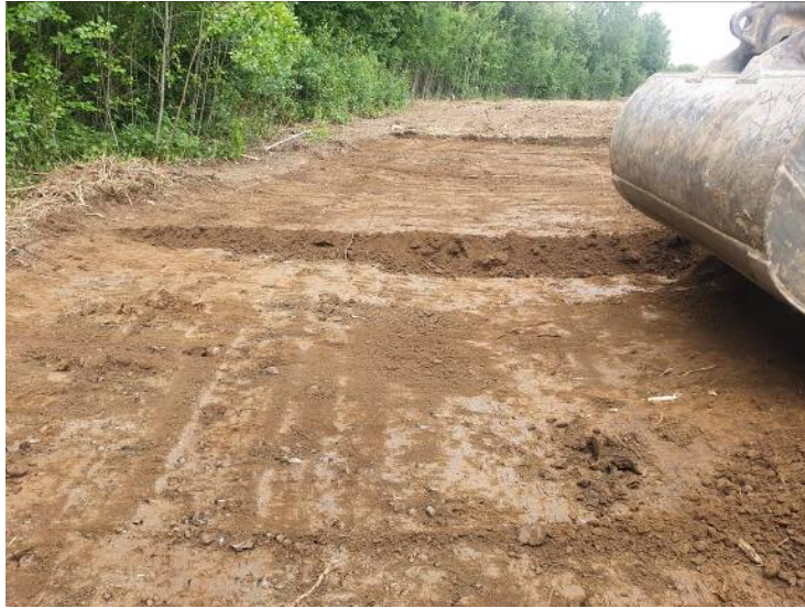
Plate 5 The start of the topsoil strip, facing north.
