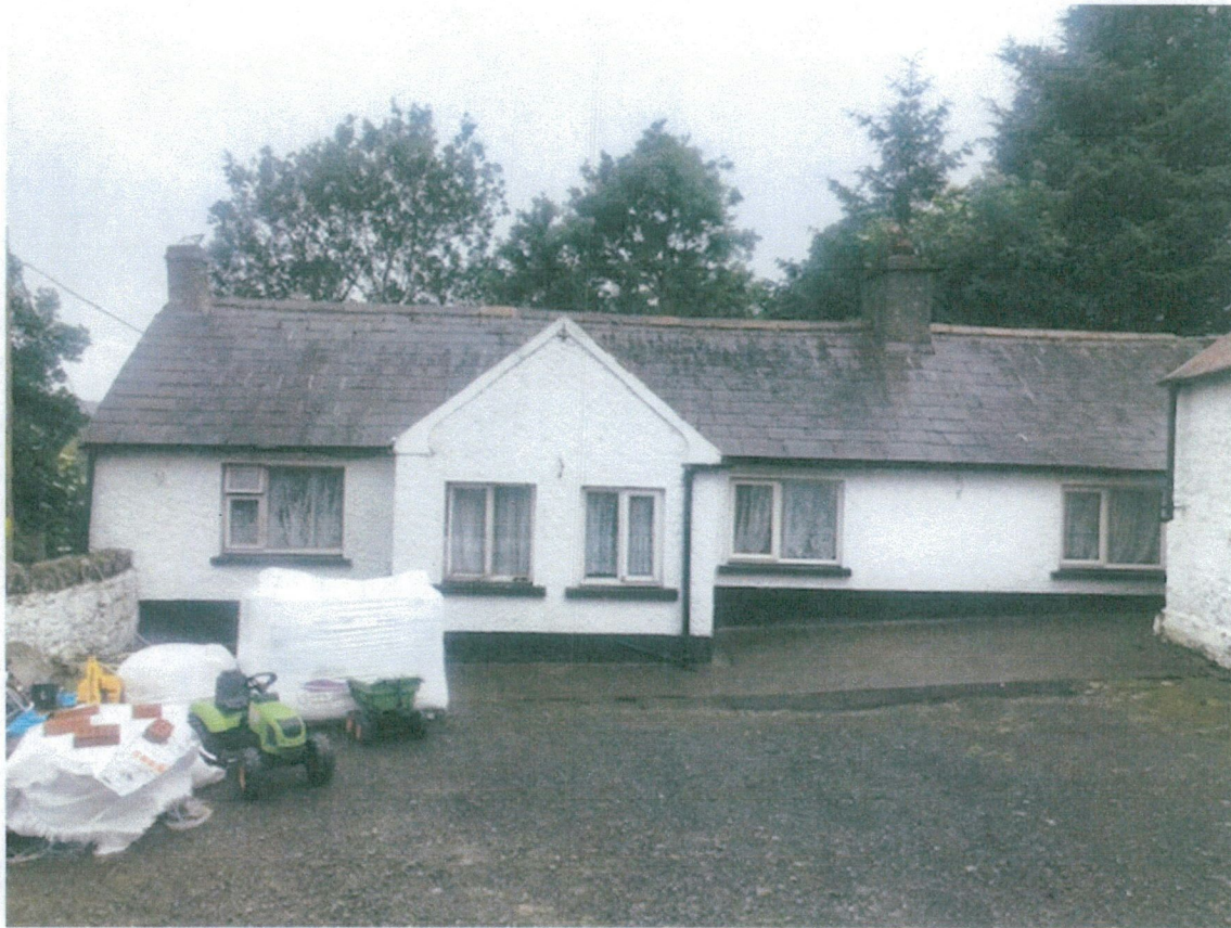
Photo 01 - Front elevation of property
