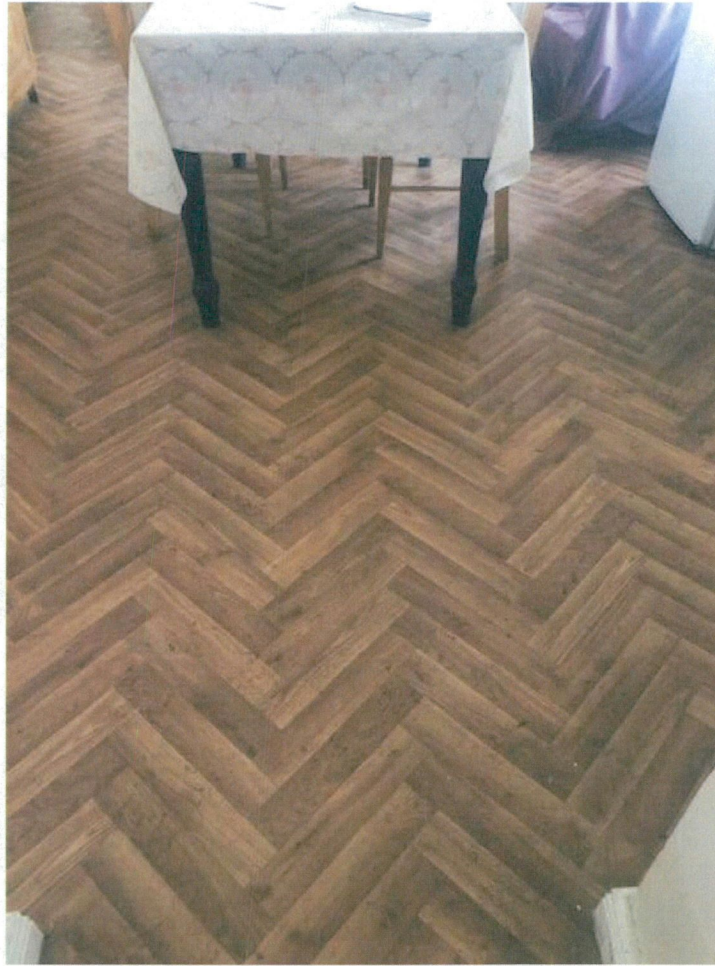
Photo 11 – Floors to kitchen
