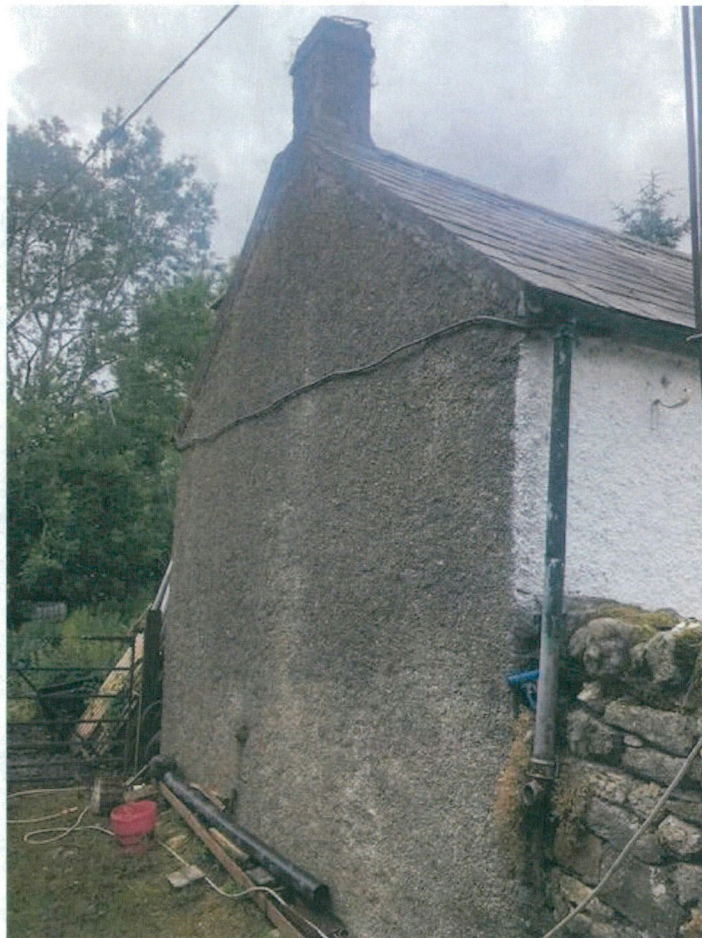
Photo 03 – South gable and chimney
