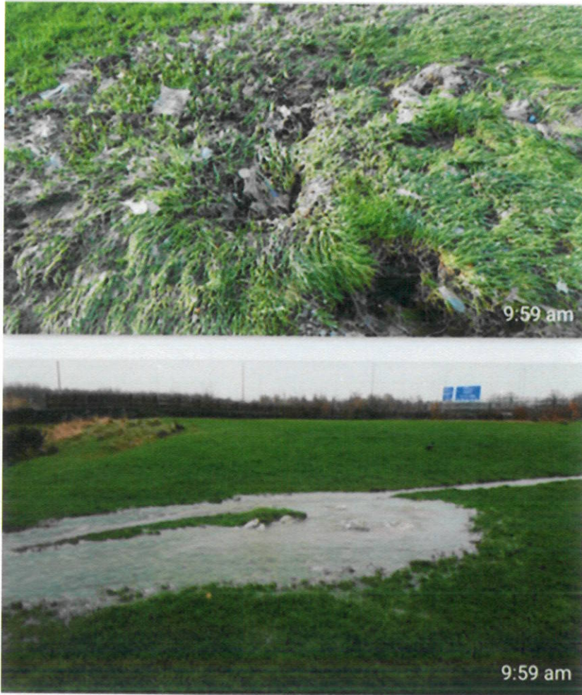
Figure 4: Compilation of Sewerage Backup within the Open Space in the Area
