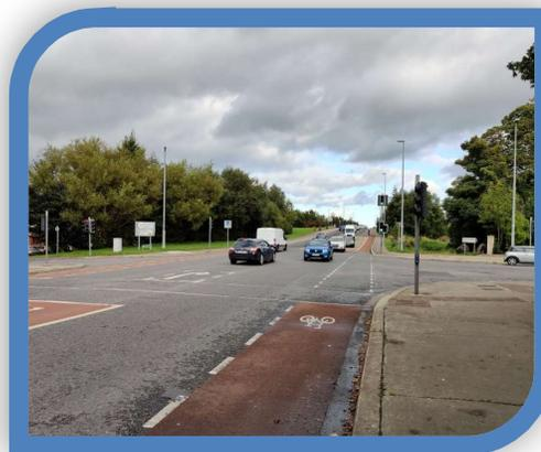
All arms of the junction include signalised pedestrian crossing facilities, in addition to dropped kerbs, tactile paving and crossing markings. The approaches to the junction from Firhouse Road and Ballycullen Road also feature advanced stop lines and storage space for cyclists. Advisory cycle lanes are also present through the junction on Firhouse Road. The Ballycullen Road arm of the junction also includes an advisory cycle lanes which accommodates right-turning cyclists.
