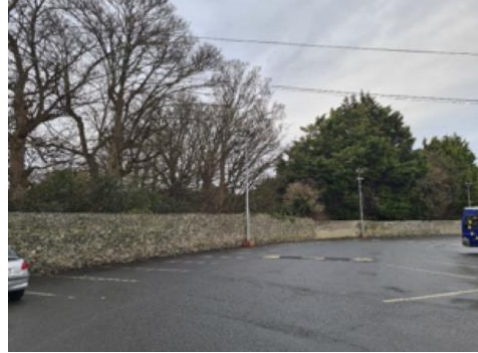
Fig. 2 Boundary wall of Inn car park with mature broadleaved trees shown.
