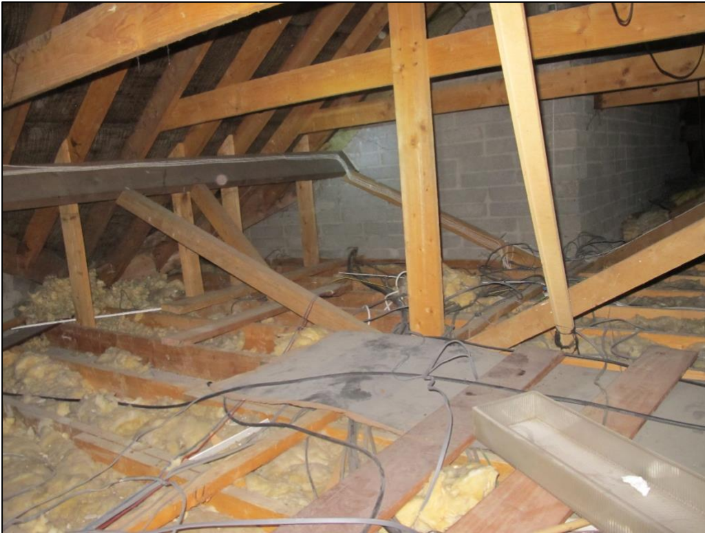
Plate 11. Front attic of two story modern building.
