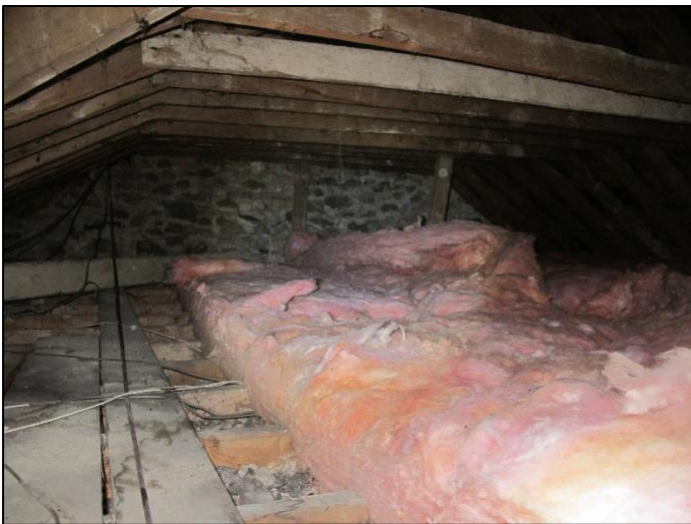
Plate 6. Firhouse Inn attic, showing return at eastern end
