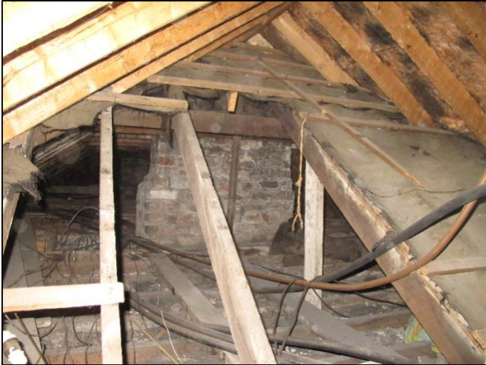
Plate 5. Firhouse Inn attic showing middle attic
