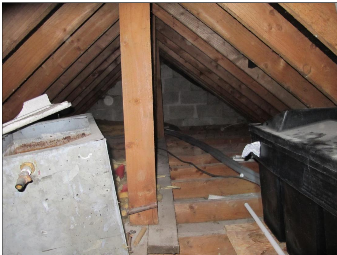
Plate 8. Interior attic of cottage (rear attic)
