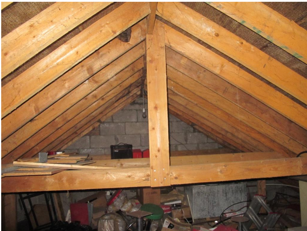
Plate 12. Rear attic of two story modern building.
