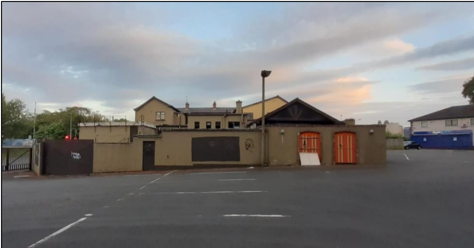
Plate 2. Rear of Firhouse Inn. View to south
