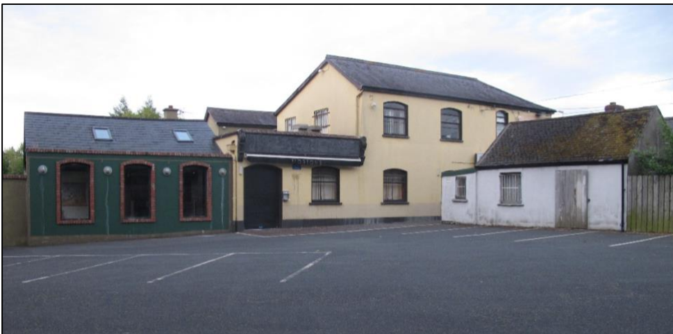
Plate 3. Rear of Firhouse Inn and cottage. View to east.
