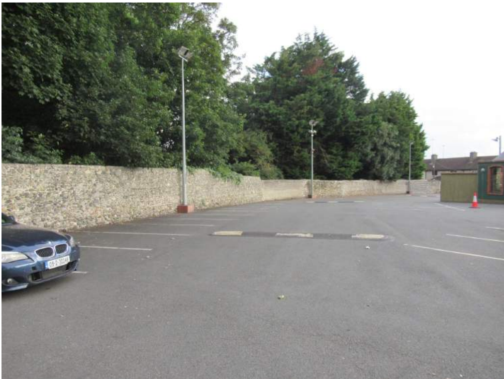
Plate No. 7. General view showing the rubble stone boundary wall at the west side of the development site.
