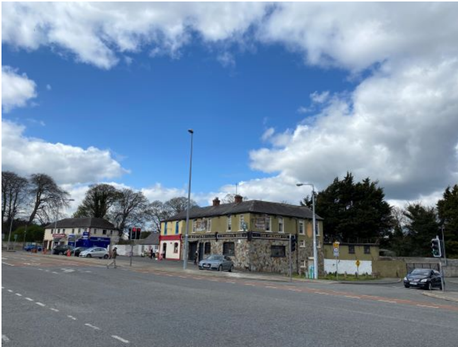
Plate 1 View of site from south east
