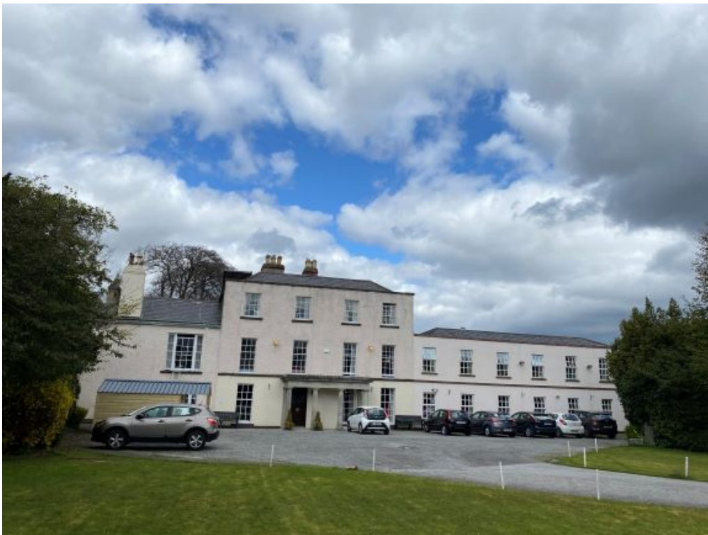
Plate 4 South facing façade of Sally Park (DU022-103---)
