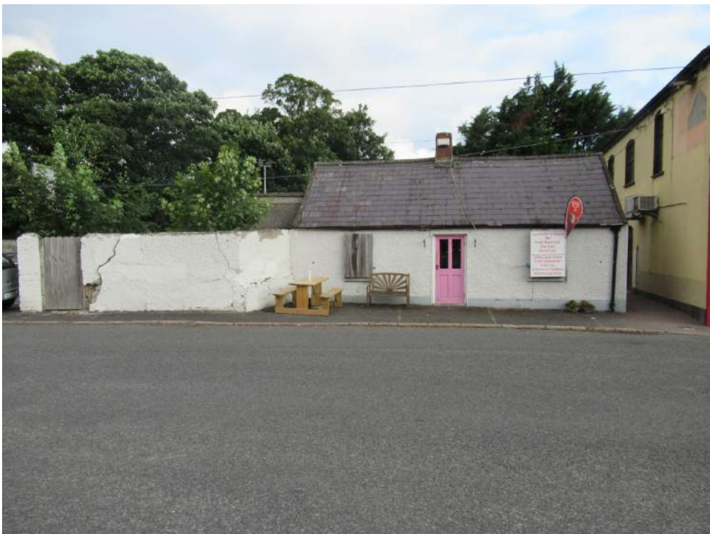
Plate No. 5. Primary south elevation of the cottage and its yard.
