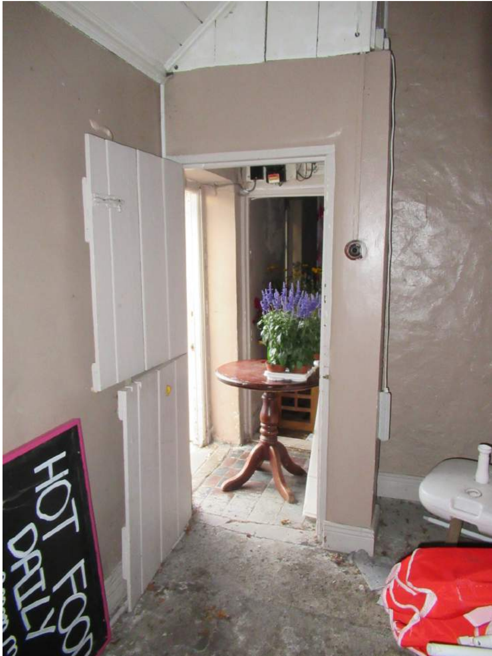
Plate No. 10. Internal view looking towards the entry from the east room in the cottage. The entry is paved with red and black terra cotta tiles, commonly used during the late 19 th and early 20 th centuries.
