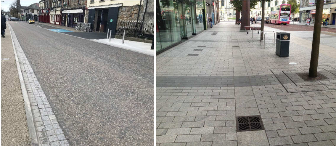
Figure 41. HRA asphalt used to distinguish vehicular surfaces at ground floor level; permeably detailed golden coloured granite elsewhere in the public open space, including to tactile hazard warning surfaces, kerbs, footpaths, and shared space circulation areas
