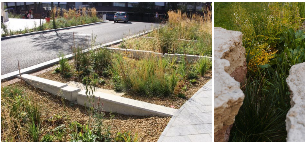
Figure 53. Details such as kerb cuts and check-dams can deal with a gently sloping site and still provide 'rain garden' type functions; providing flat-topped boulders in a rain garden provides an informal opportunity for play as stepping stones
