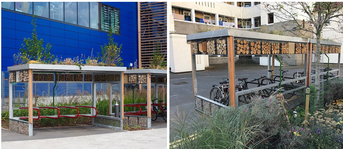
Figure 43. Open sided green roof cycle shelters with Sheffield type locking stands provided in the public amenity open space and in the creche secure external area
