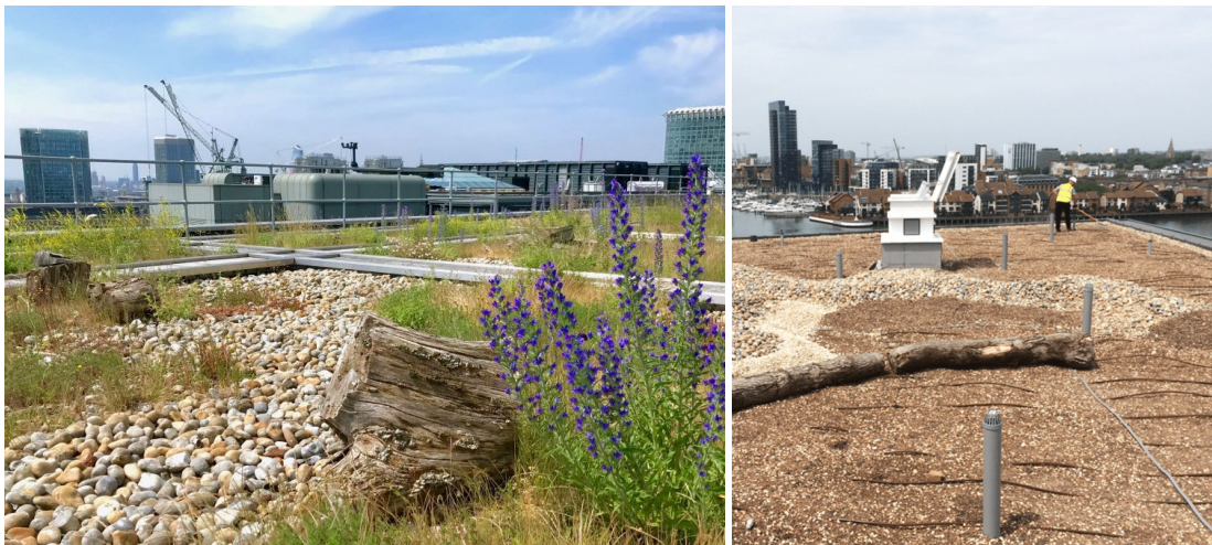
Figure 50. Biodiverse roof with mounded topography, deadwood piles, gravel areas and larger-depth substrate amenity planting
