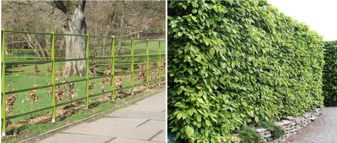
Figure 37. Painted estate type railing to 1.20m ht, with a clipped formal hedgerow of naturalised Hornbeam behind it, to buffer the amenity space from the noisy public road
