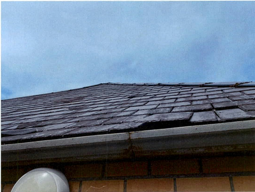
Photo 13: Detail of roof condition, south elevation
