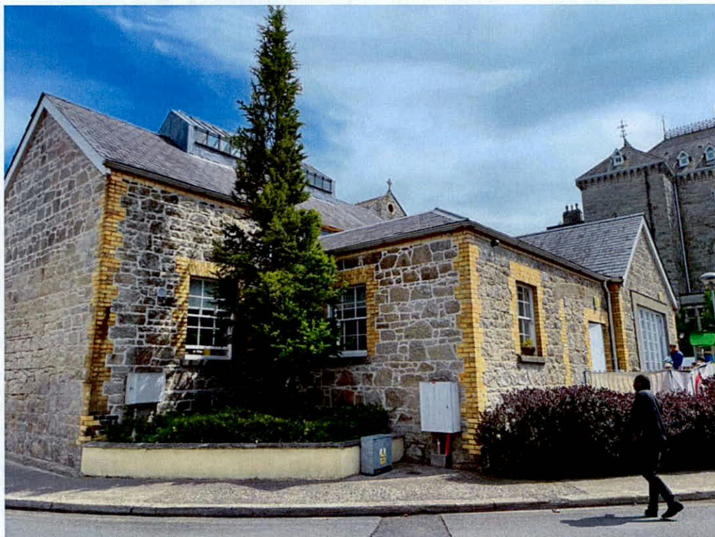
Photo 6: North-west oblique view from roadway
