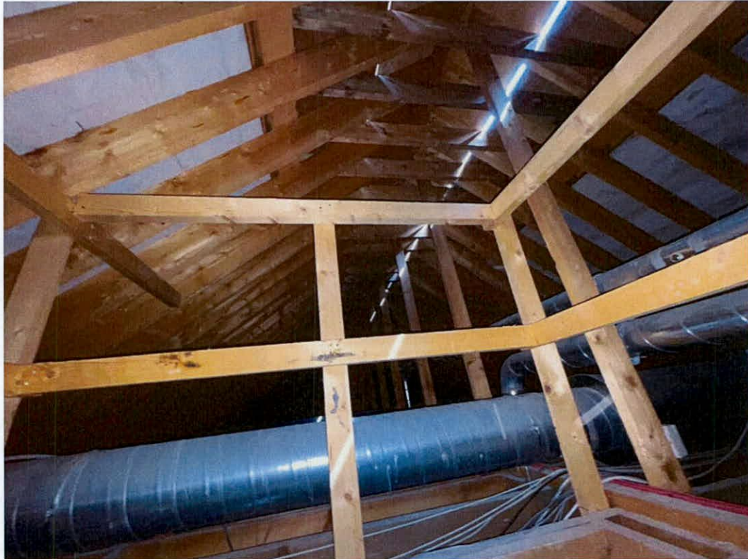
Photo 24: Attic space over central roof section/staff room & sleep room
