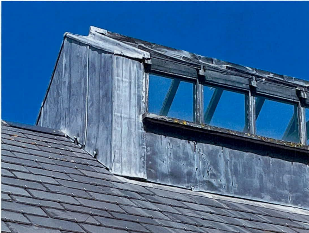
Photo 15: Detail of typical condition of roof lanterns
