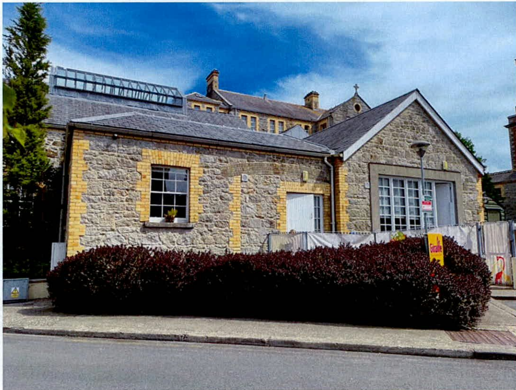
Photo 5: West elevation view from roadway
