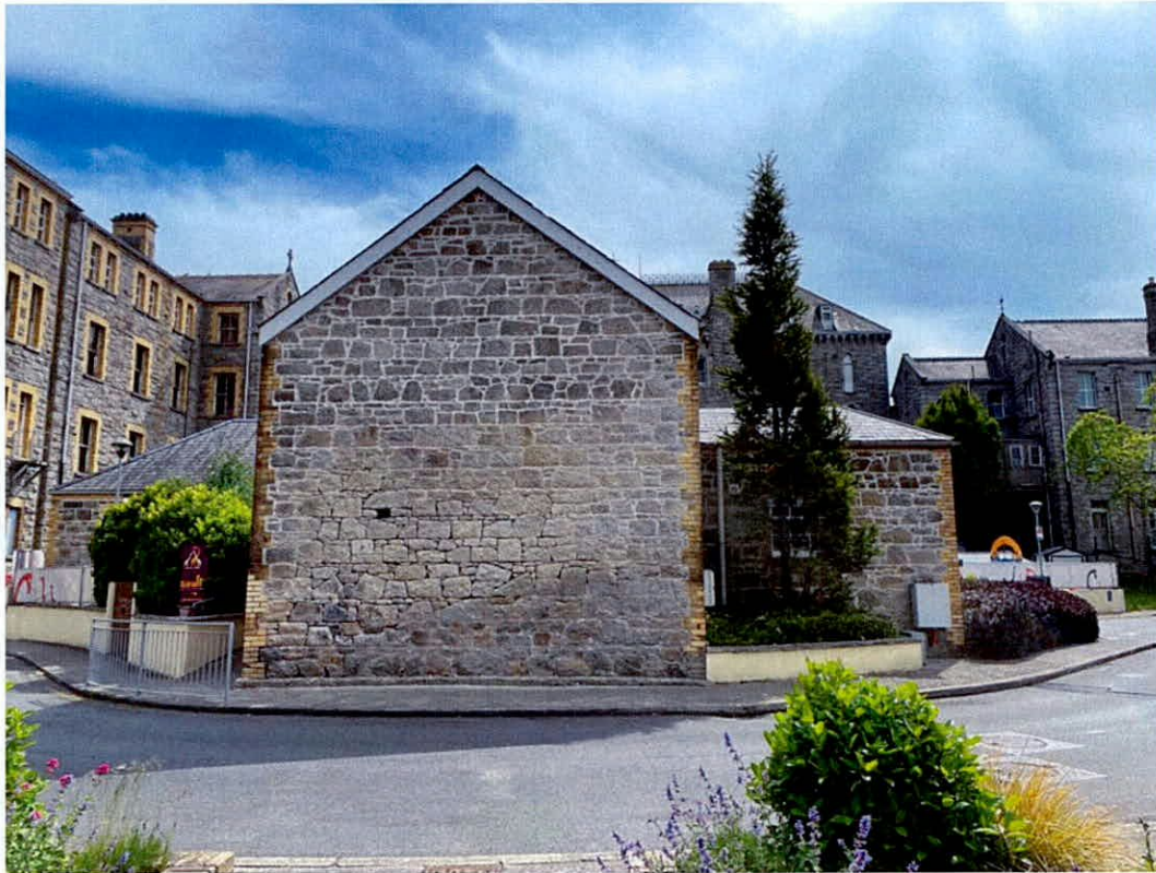
Photo 7: North elevation gable
