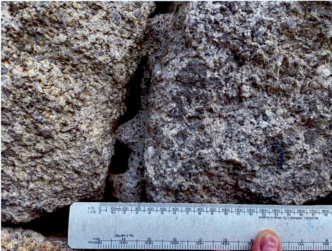
Photo 9: Detail of extant historic mortar to bedding joint to north elevation
