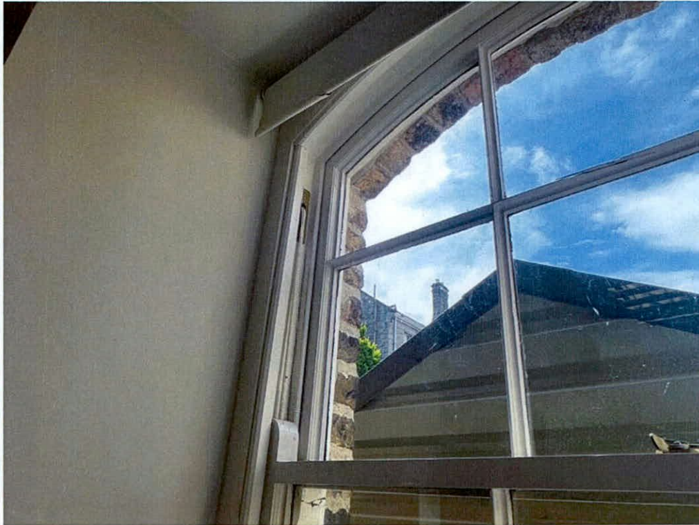
Photo 19: Sample internal detail of typical reproduction sash window joinery
