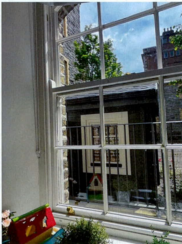
Photo 20: Sample internal detail of typical reproduction sash window joinery
