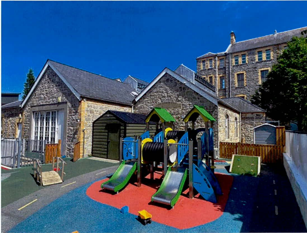
Photo 1: West elevation view from playground
