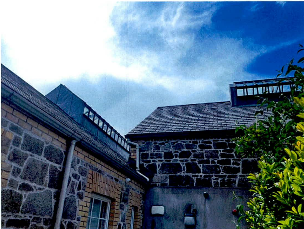
Photo 10: Detail of roof lanterns from east entrance area
