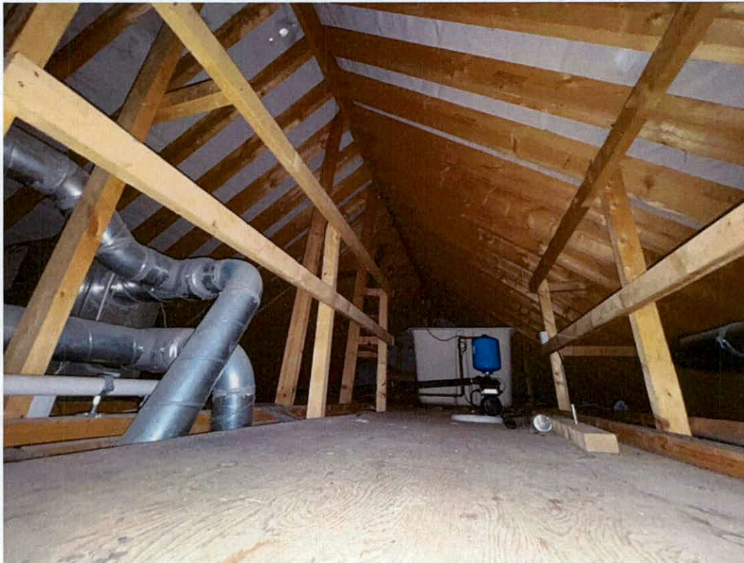
Photo 23: Attic space over central roof section/staff room & sleep room
