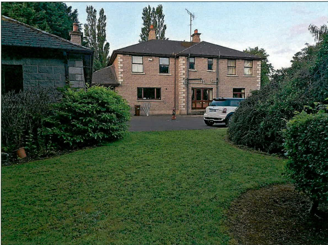
Plate 5. The adjoining Oakvale House contains a Soprano pipistrelle maternity roost.
