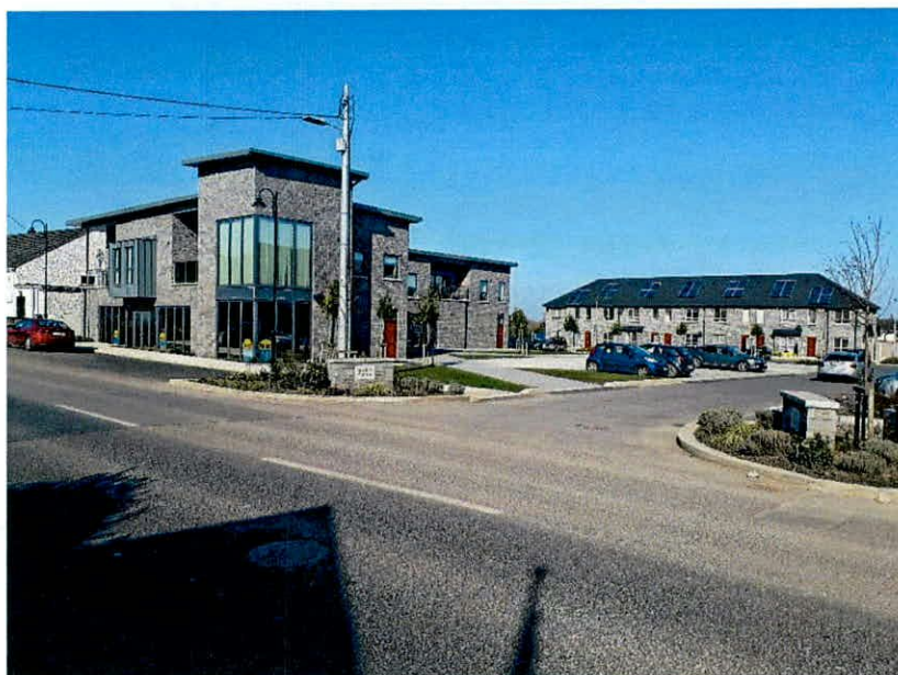
Plate 2 Adjacent Existing Development on Towerhouse site
